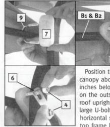
Position the assembled canopy about three inches below the roof
